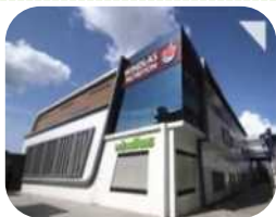
Dehradun Plant 1 commenced operations in 2001
