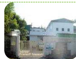
Dehradun Plant 3 commenced operations in 2018
