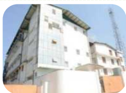
Dehradun Plant 2 commenced operations in 2014
